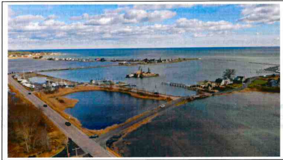
The picture above was taken at approximately 12:30pm on November 17, 2020. This was a 12.1 ft. Spring or "King" tide. Note the "pond" in the center of the lot that enters the facility from the drainage swale located in the middle of the seawall. The next Spring tide will occur on Monday, January 23, 2023, where Rye Harbor will see a 13.06' tide.
